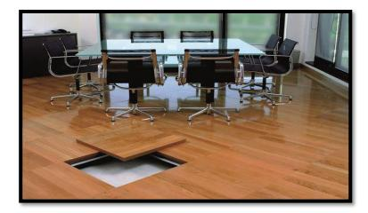
3.Command Centers and Control Rooms: In command centers and control rooms, raised floor solutions are used to accommodate large cabling infrastructure and offer easy access for repairs and maintenance.
